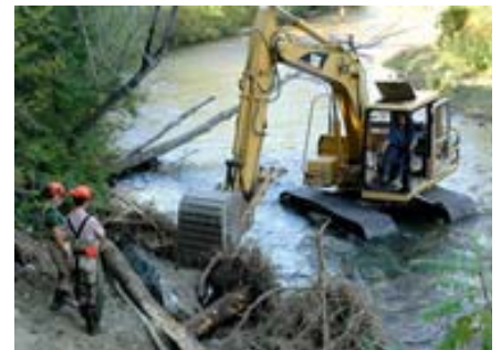
Bank stabilization project
